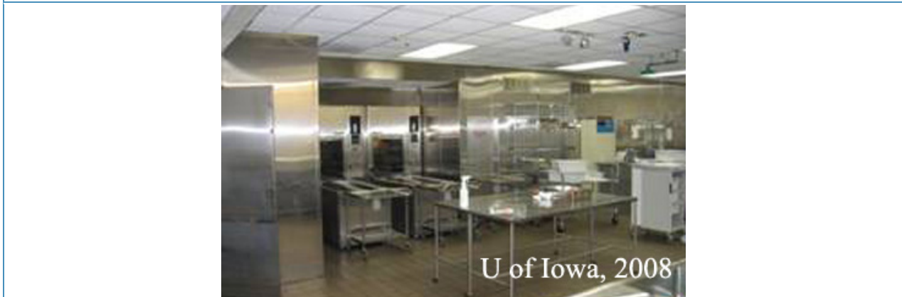
Figure 1C: Another view of the decontamination room showing the large automated washing machines that connect to the clean side of the facility.
